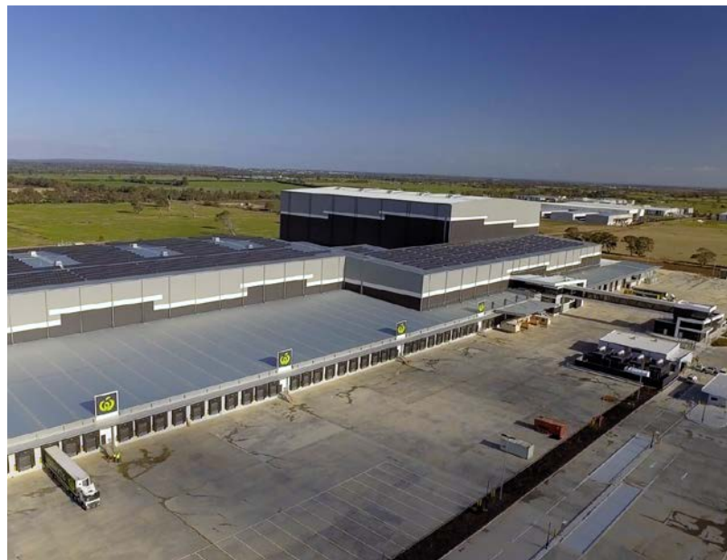
Melbourne South Regional Distribution Centre, VIC.
